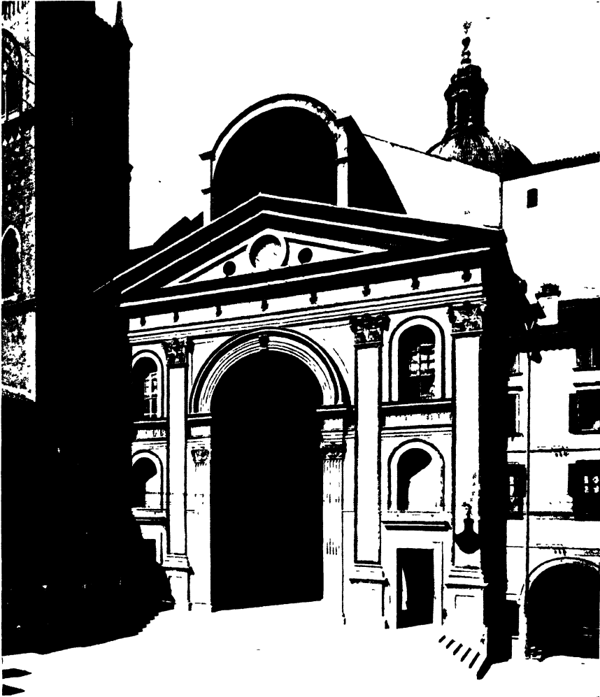
158. A Renaissance Church: S. Andrea in Mantua. Designed by ALBERTI about 1460
